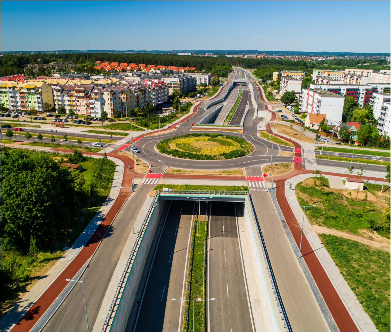
Bridge structures and retaining walls on the Trasa Niepodległości in Białystok, Poland
